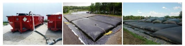
Figure 2. Multiple sizes of Geotubes enables customized dewatering applications ranging from roll-off bins (left), single-layer cells (centre) and stacked configurations that can be several layers high.
