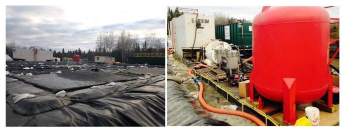
Figure 10. A Geotube dewatering cell (left) designed to dewater and contain contaminated sediments. A carbon filter system (right) was installed to remove hydrocarbons from the Geotube filtrate.
