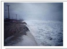
Geotube® geocontainment technology in action. Hurricane force winds and water eroded away the sand in front of the unit, but it held fast.
