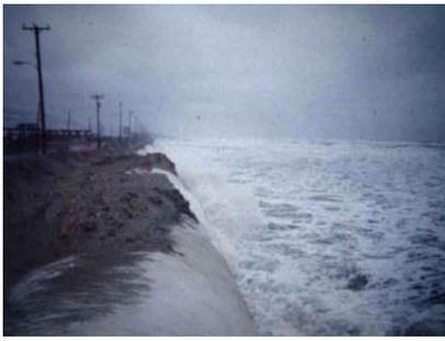
*Geotube® geocontainment technology in action. Hurricane force winds and water eroded away the sand in front of the unit, but it held fast.*
