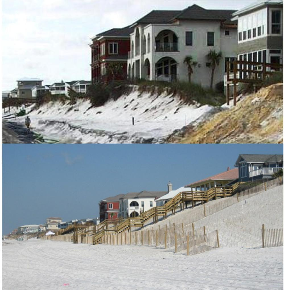
*Before and After: A Florida beachfront so damaged by recent hurricanes that a Geotube® unit was needed to save homes, and (after) recreation following the installation of Geotube® geocontainment technology.*
