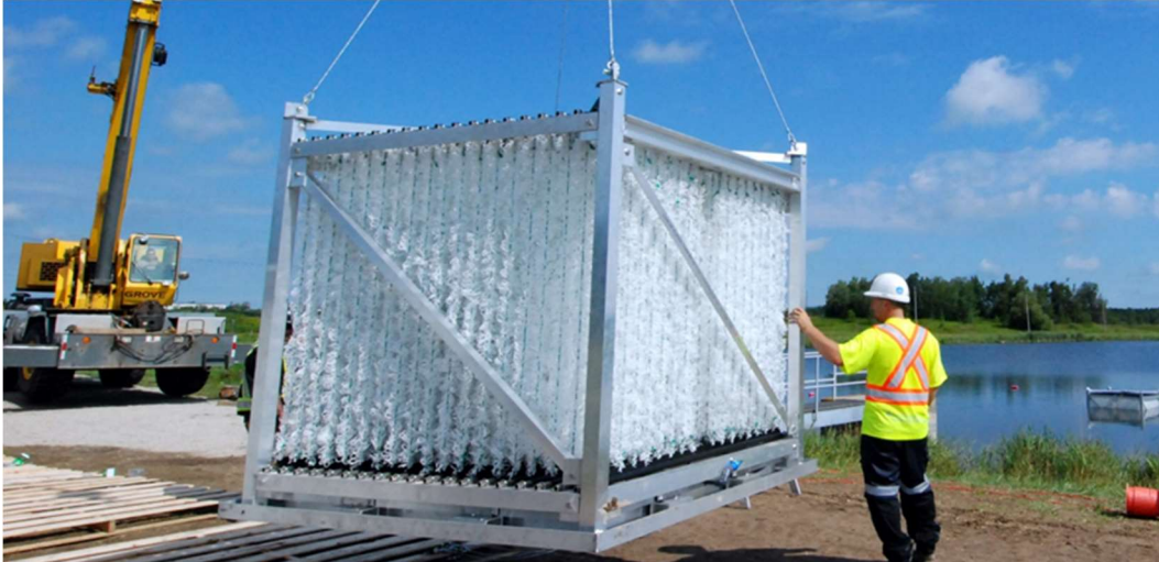
FIGURE 9. BIOCORD REACTORS CAN BE SHIPPED TO SITE FULLY ASSEMBLED AND INSTALLED IN JUST A FEW DAYS, WHILE THE LAGOON REMAINS IN OPERATION (FILE PHOTO).
