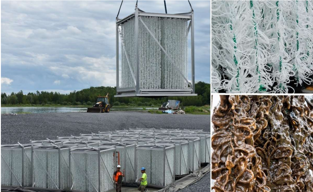
FIGURE 1. BIOCORD MEDIA IS A CONDOMINIUM FOR BACTERIA THAT INCREASES THE CONCENTRATION OF MICROBES TO IMPROVE COLD-WEATHER REMOVAL OF BOD AND AMMONIA
