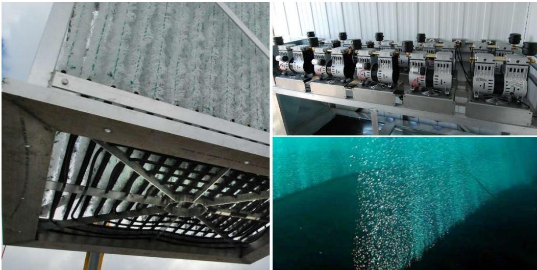
FIGURE 11. FILE PHOTO SHOWIING FINE-BUBBLE AERATION TUBING INTEGRATED INTO THE BASE OF THE REACTOR. AIR IS SUPPLIED BY LOW-ENERGY COMPRESSORS, INSTEAD OF BLOWERS.
