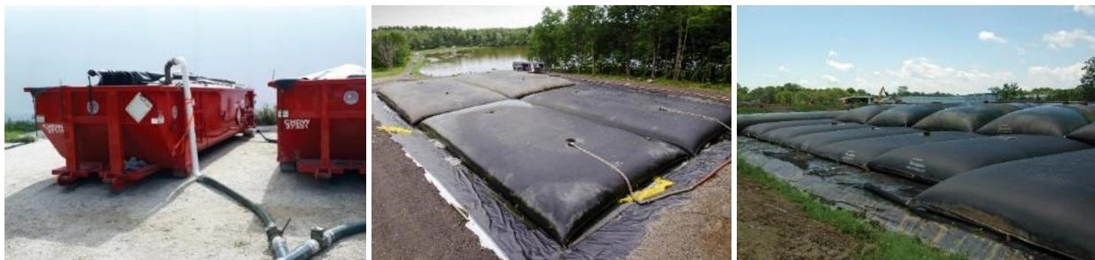
Figure 2. Multiple sizes of Geotubes enables customized dewatering applications ranging from roll-off bins (left), single-layer cells (centre) and stacked configurations that can be several layers high.
