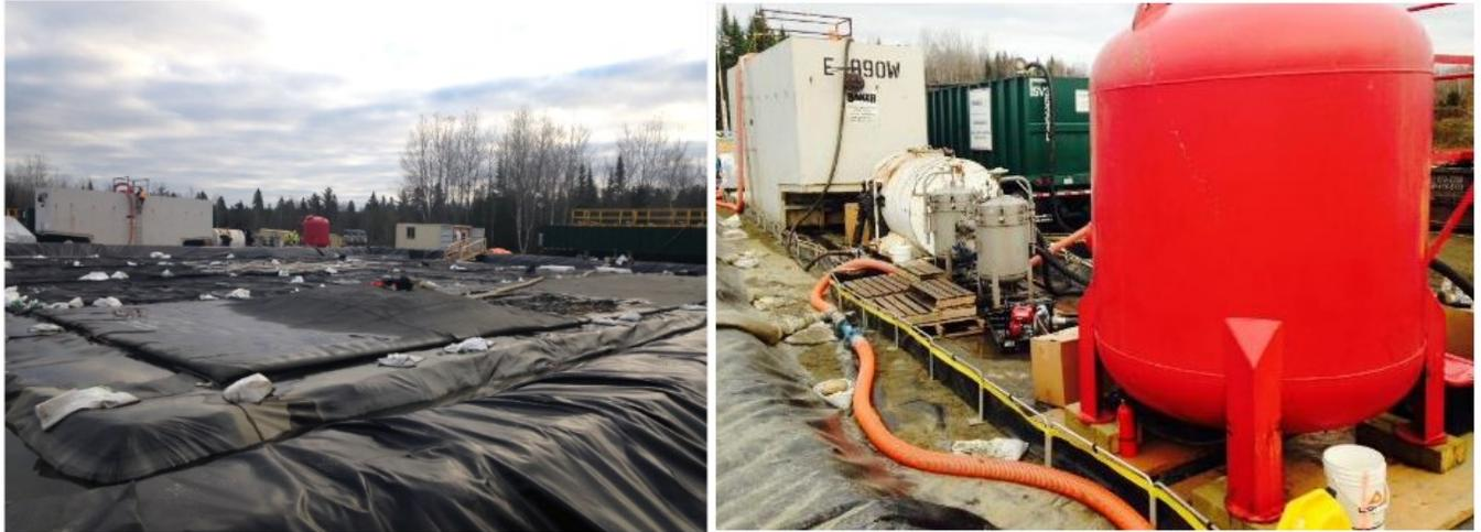
Figure 10. A Geotube dewatering cell (left) designed to dewater and contain contaminated sediments. A carbon filter system (right) was installed to remove hydrocarbons from the Geotube filtrate.
