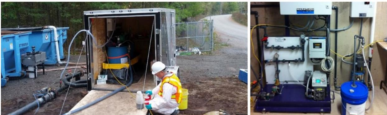
Figure 6. A small trailer (left) contained the polymer dosing system and flocculator for the pilot test. The VEPAS (right) incorporates few components and provides simple polymer activation and dosing.
