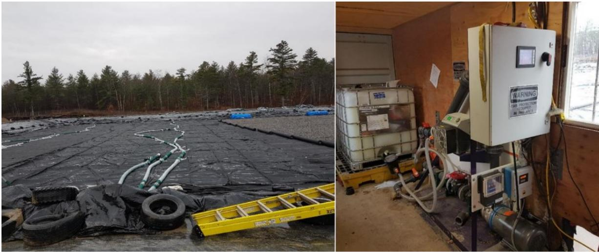
Figure 7. The full-scale demonstration project included a lined dewatering cell that held seven Geotubes, 120 ft circumference by 186 feet in length (left.) A larger, containerized polymer system was also brought to site. Over the duration of the demonstration project, the crew dewatered 24,905.5 m<sup>3</sup> (32,575 yd<sup>3</sup>) of contaminated sediments, which corresponds to 1,789.07 bone dry tonnes (1,972.11 bone dry tons).
