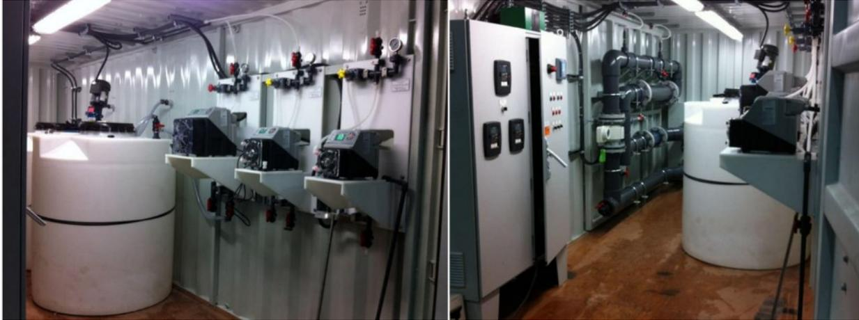
Figure 9. The components of the water treatment system included a mixing tank and peristaltic pumps (left) and a control panel, flocculator and flow meters (right).
