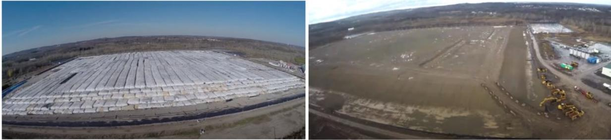
Figure 11. The Geotube dewatering cell at Onondaga Lake is stacked up to five layers high and occupies about 22 hectares. The image on the right shows the cell once capping was complete and prior to adding vegetation.
