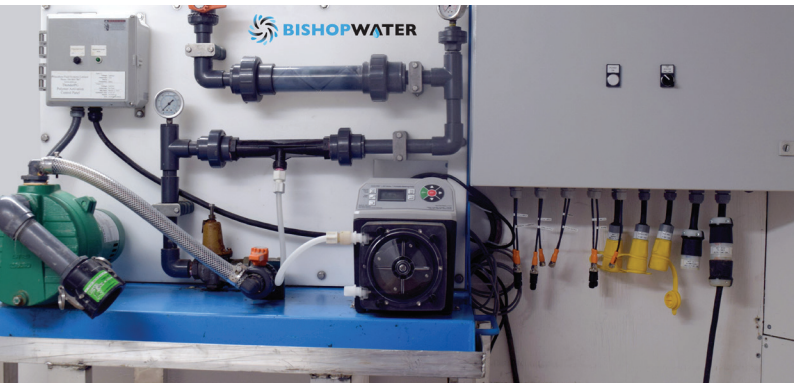
Figure 2. Example of Bishop Water Vepas 100 Chemical Injection Unit
