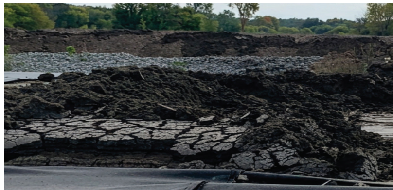
Figure 3. The dewatering and subsequent consolidation of materials within the Geotube® allows for a more efficient solids management solution.
