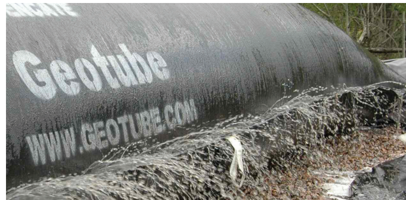
Figure 1. Geotube® unit discharging effluent. The Geotube® uses specially-engineered fabric to capture solids within, while allowing the release of clear effluent often at a state of quality ready for release back into waterbodies.
