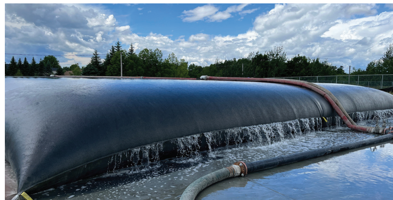
Representative Geotube® dewatering system in operation
