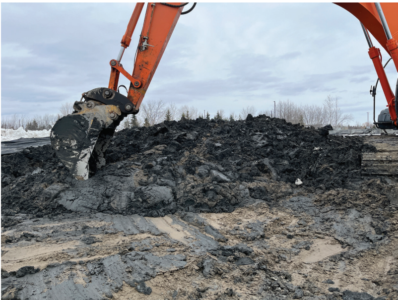
Representative sediment disposal operation
