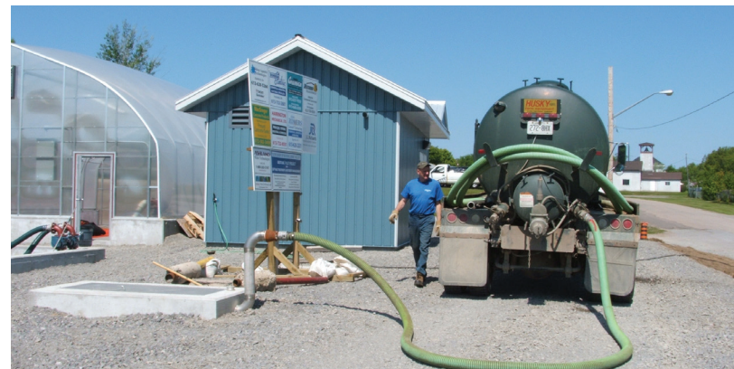
Septage haulers can discharge trucks into an underground 10,000-gal tank, which is pumped into Geotubes when full.
