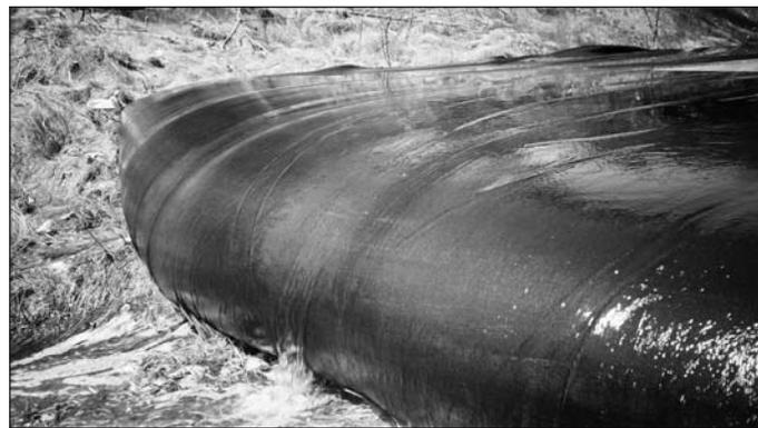
Clean filtrate flows from Geotube® while filling.
