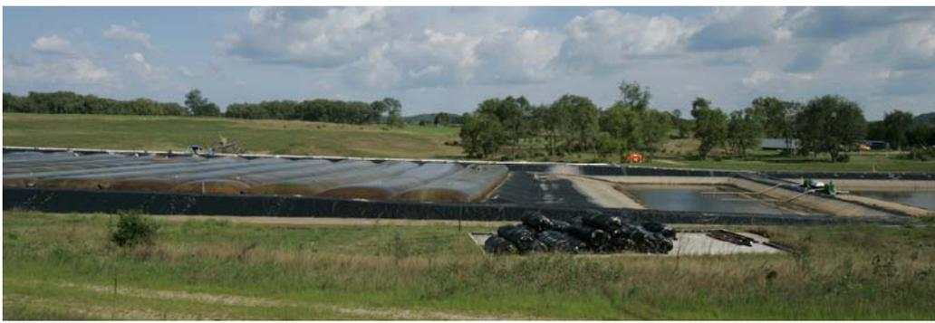
*Geotube® containers provide permanent safe landfill storage for heavy metals with filtrate providing safe water for irrigation or option of returning filtrate to Geotube® containers for additional filtering.*
