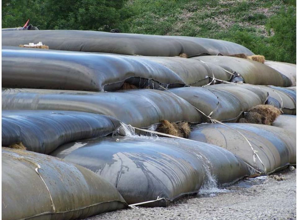
*Geotube® containers yearly stacked 4 to 6 layers high over a five year period provided dewatering, containment and removal of PCBs at the headwaters of the Fox River, Little Lake Butte des Morts.*
