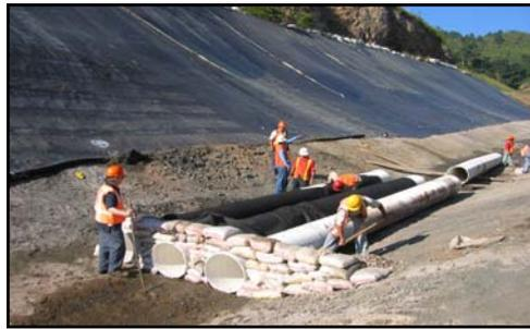
Installation & bedding of HDPE drainage pipe at base
