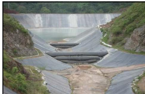
Drainage raceways leading into tailings lagoon
