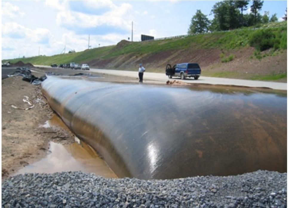
*Geotube® dewatering technology has been successfully used for tailings treatment in a variety of applications. In this project, Geotube® dewatering technology was used to help treat acid tailings from a mine. After treatment, water quality was good enough to release back into streams.*
