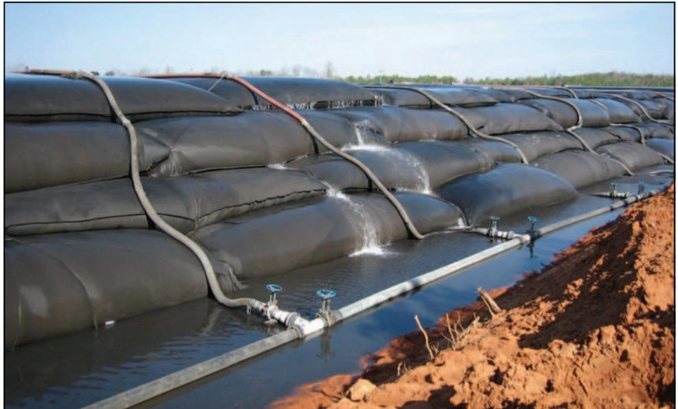
*Geotube<sup>®</sup> technology, perfectly suited to both dewater and contain materials, solved the slurry waste disposal issues facing the North River Mine. This large-scale project involved 3 bag fields, 240 Geotube<sup>®</sup> containers, and 200,000 cubic yards of coal slurry waste being pumped and dewatered.*
