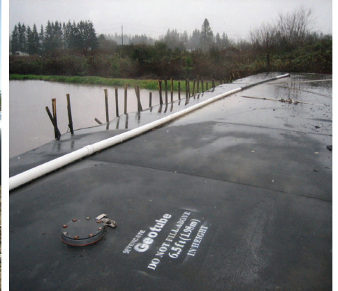
Figure 3. Filled Geotube® unit next to clean lagoon.
