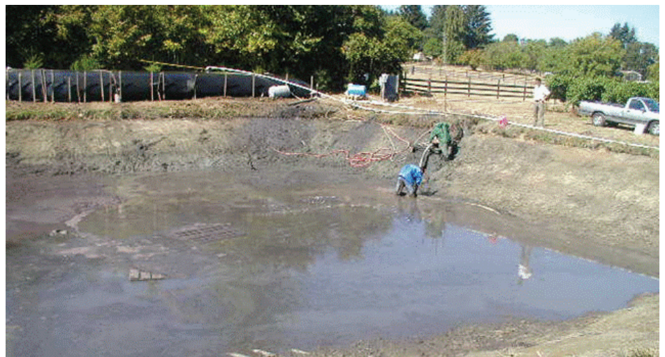
Figure 1. Cleaning the lagoon with Geotube® unit in the background.
