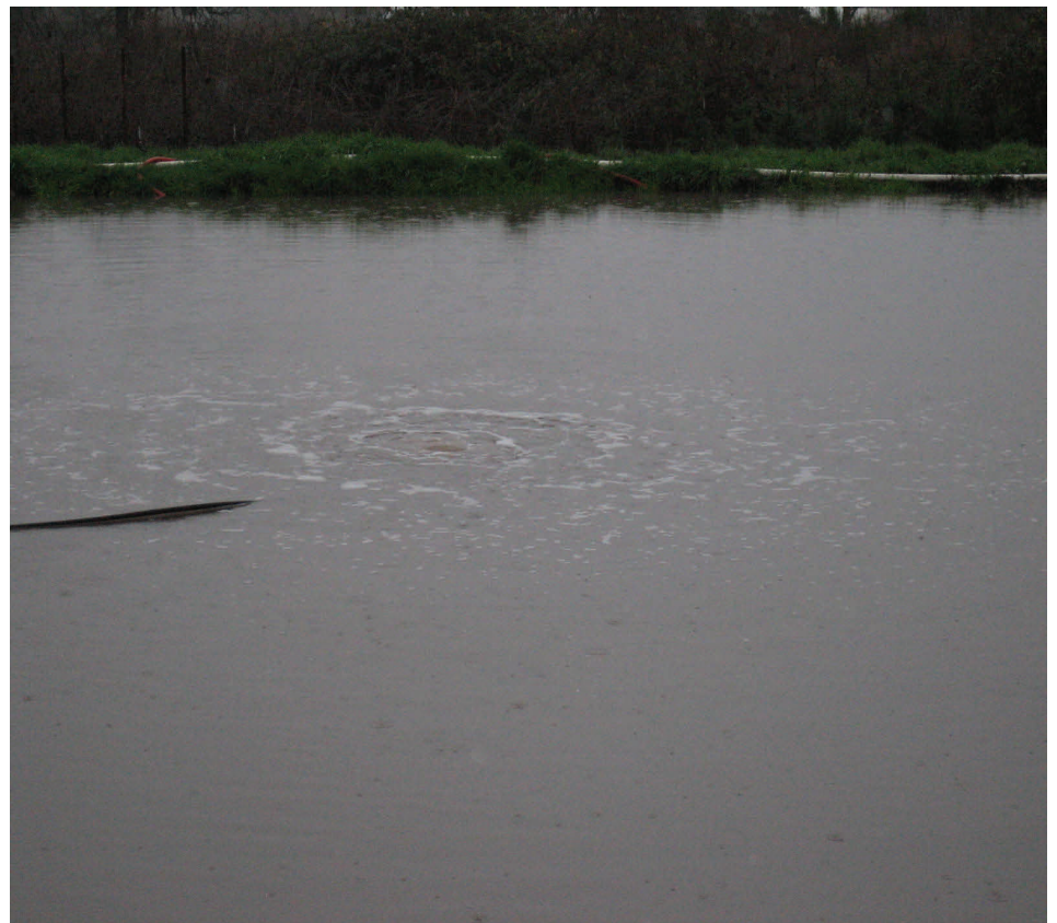
Figure 4. Aeration system providing aerobic digestion to the clean lagoon.
