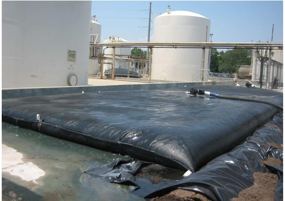
*By using custom-sized Geotube® containers designed to fit into open spaces available on the job site, Arizona Chemical was able to dewater more than 1,000 tons of sludge in less than two weeks. This is half the time of other dewatering methods, plus it was 38% more cost-efficient.*
