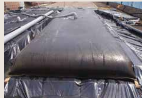
Dewatering of oil sludge
