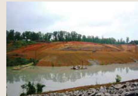
Reclaimed site after dewatering
