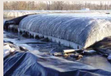
Dewatering under winter conditions
