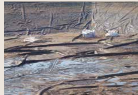
Pond empty for HDPE liner repair
