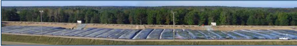
Geotube® dewatering technology can be used for large and small projects. The individual Geotube® units can be as long as 200 feet with a circumference up to 65 feet. Units can even be stacked if space is at a premium.
