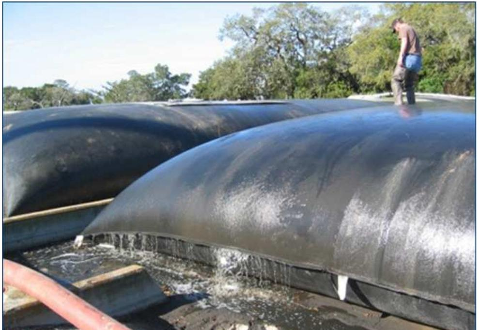
*In Jekyll Island, GA, Geotube® dewatering containers were used to provide a fast way to remove more than 400,000 gallons of sludge from digesters. The Geotube® containers fit into the facility's existing drying beds and made the process simple.*
