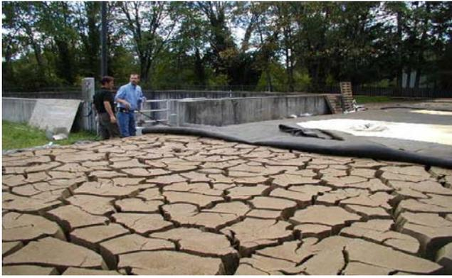
*Dewatered alum sludge in Grants Pass, OR shows the efficiency of Geotube® dewatering technology.*
