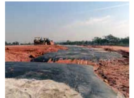
Capping a Geotube® dewatering cell
