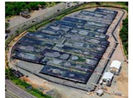
One of the Geotube® dewatering cells
