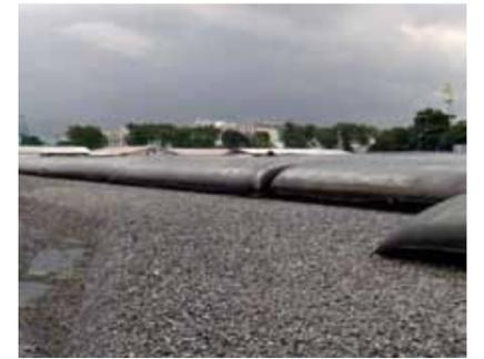
Geotube® dewatering platform
