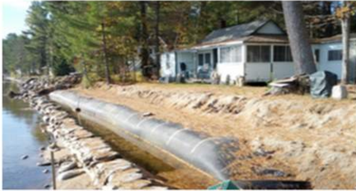
Geotube® Installation in Fall of 2013
