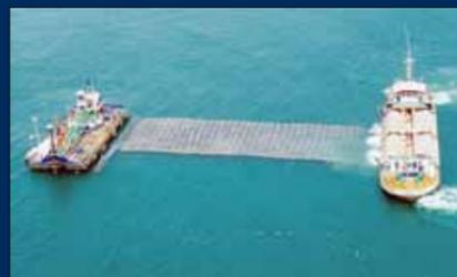
TenCate's Mirafi® woven geotextiles are used as filters beneath rock-fill breakwaters and bed protection works to prevent the erosion of the foundation soil. TenCate's Geotube® and Geocontainer® geocontainment materials are used for the cores of breakwaters providing mass-gravity, stable structures.
